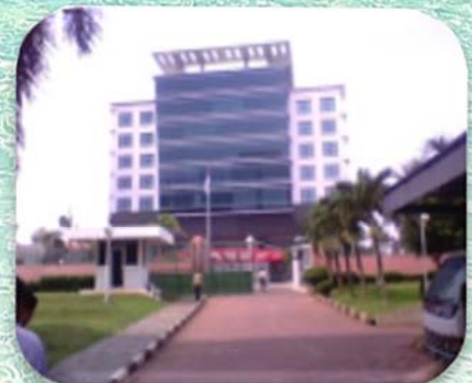
Data Center BRI Ragunan Project
