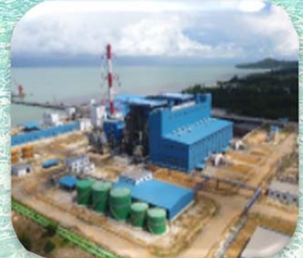
Project PLTU Bengkayang Kaltim
